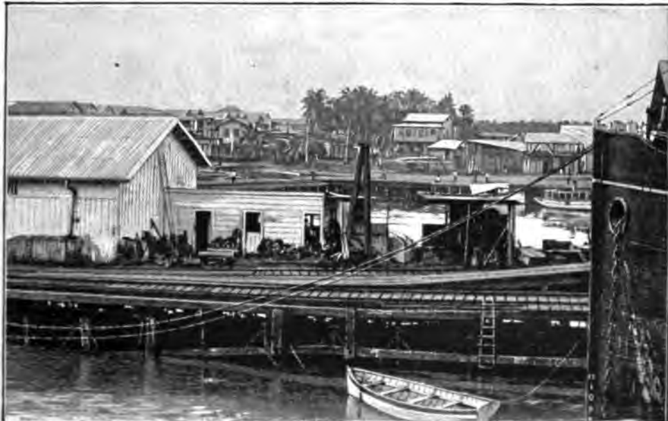
WHARF AT COLON.
