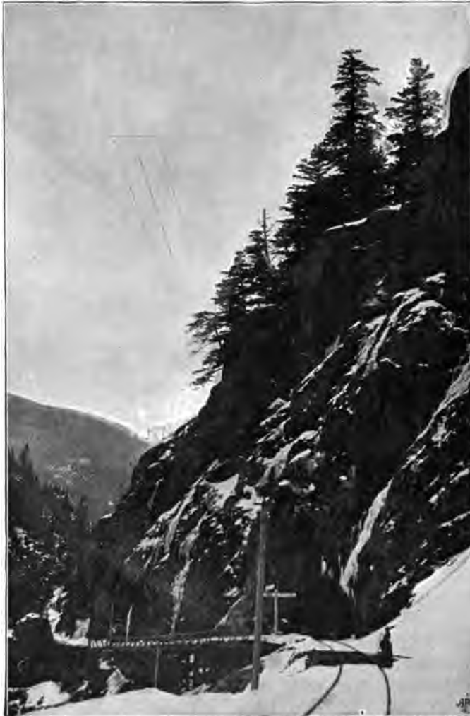
WAGON ROAD ROUND A BLUFF IN THE MOUNTAINS—RAILWAY TRACK THROUGH IT.
